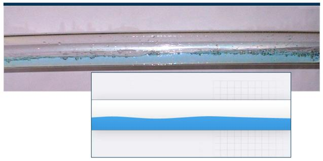
Under light rainfall, the systems are going to run in what is termed gravity flow. There are air and water in the pipe and as water finds its own level, it runs to the main vertical stack out of the system.
