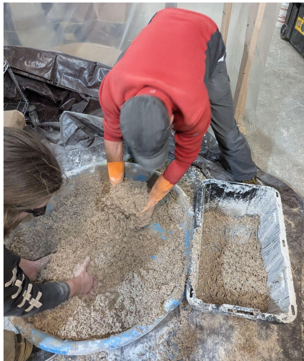
Hemp-lime 3-part mix: hemp hurd, lime-based binder, and water
