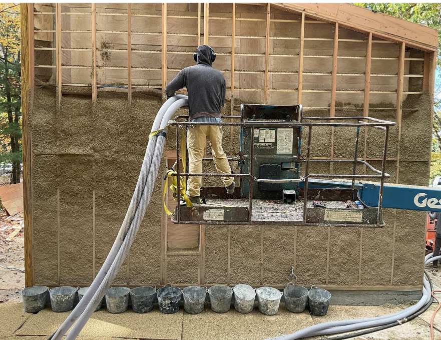
Spray-applied hemp-lime in an exterior-stud wall
