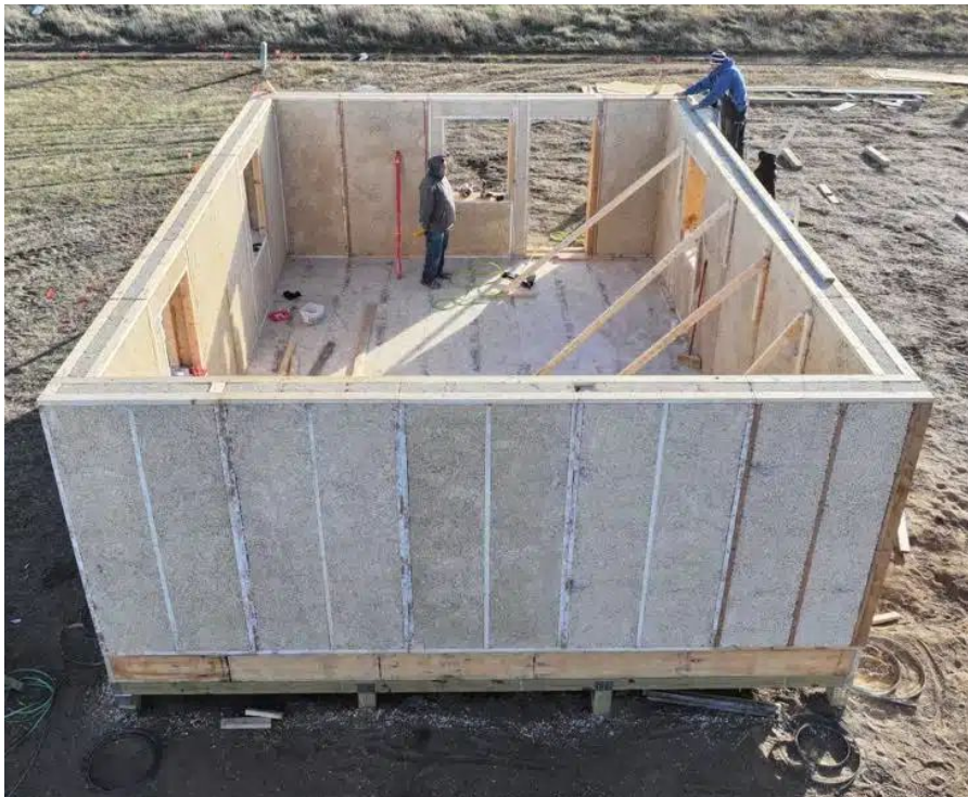
Pre-fabricated hemp-lime panels erected on-site
