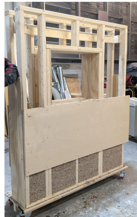
Hemp-lime double framed wall, hand-tamped with slip form
