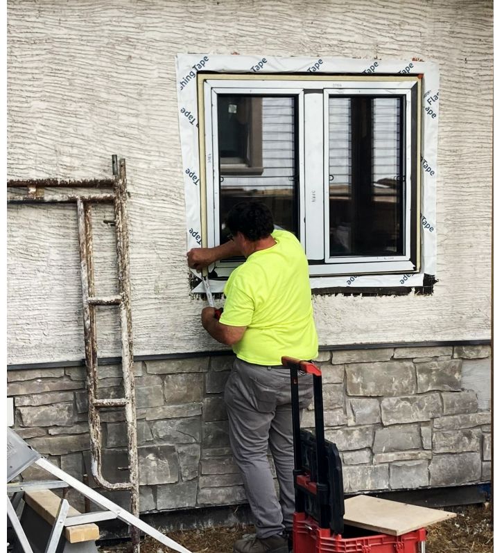
Flashing, trim, and plaster scratch coat
