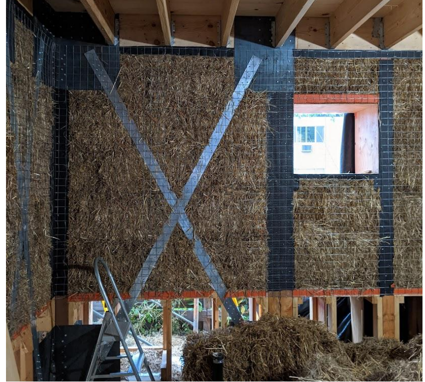
Wire mesh and lateral 'x' bracing at posts
