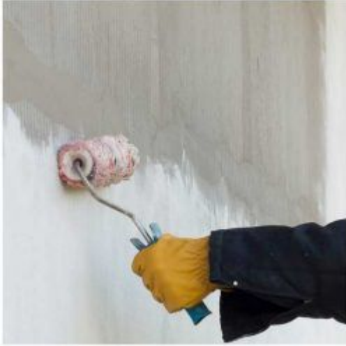
Roll, brush, or spray-applied silicate mineral paint
