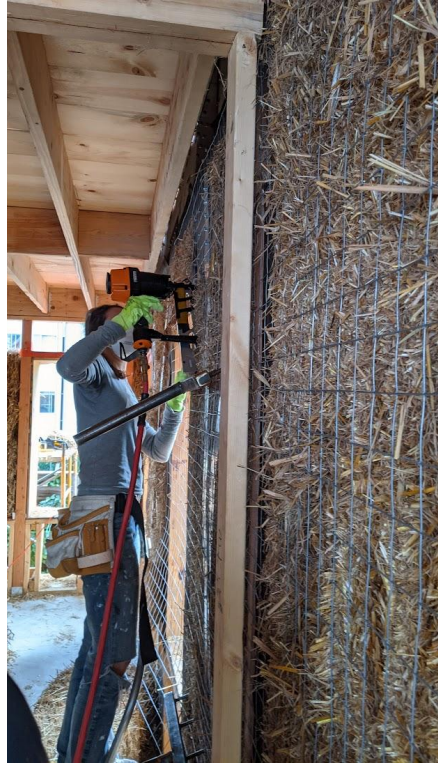
Installing wire mesh
