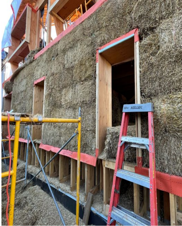
Exterior view of strawbale infill
