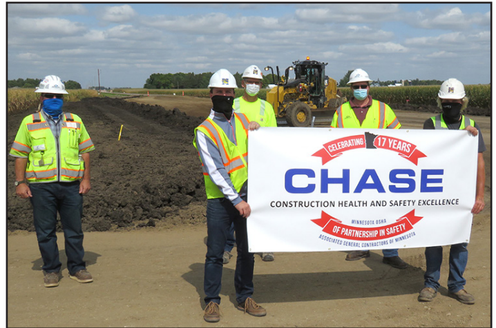
Mathiowetz Construction • Nicollet County Road 12 • Courtland Township, Minnesota
