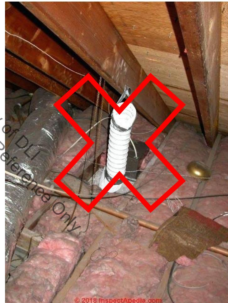
3. For all environmental air exhaust: **3 feet** from property lines; **3 feet** from operable openings into buildings for all occupancies other than Group U, and **10 feet** from mechanical air intakes. Such exhaust shall not be considered hazardous or noxious.
