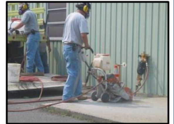
✔ Yes Engineering Controls
