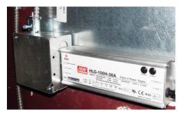
The UL standard restricts the driver output to less than 60 volts in dry applications and less than 30 volts in wet applications. To be listed, the secondary current cannot exceed 5 amps and the total power output rating must be less than 100 watts.
