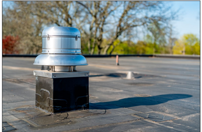
Example of curb elevated for future insulation.
