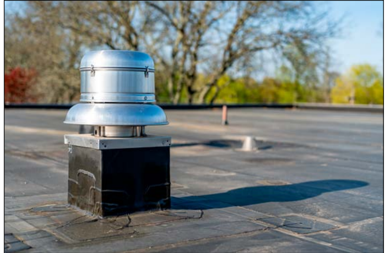
Example of curb elevated for future insulation.
