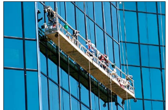
Pictured at top are boatswain's chairs. Above is a swinging scaffold.
